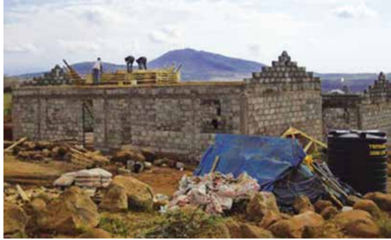
loading roof trusses
