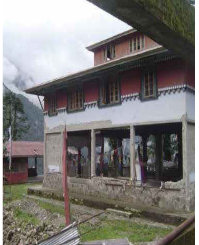
After the Earthquake of 18th September, 2011, Sikkim
